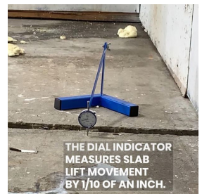
INJECTION OF AP LIFT 430 BEGINS AT THE POINT ABOVE THE LARGEST VOID.
